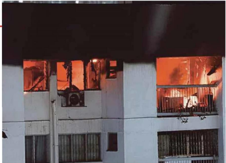
Fire engulfing units on the 17th floor of Block 70 at the Sri Sabah flats in Cheras, Kuala Lumpur, on Sunday night. BERNAMA PIC
