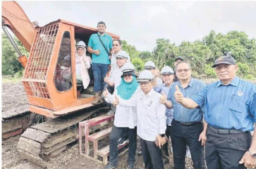
Fatimah (sitting on excavator) poses with others during the symbolic groundbreaking of the organic fertiliser plant site in Kg Kekan.
