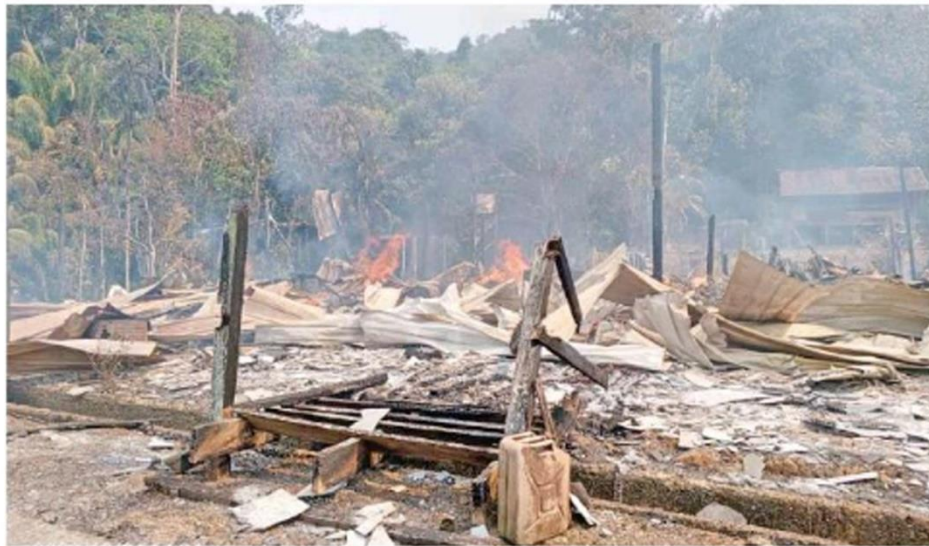
The aftermath of the fire at Rumah Sebom Bantan.
